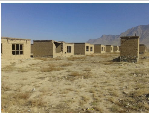
Abandoned houses, Aliceghan LAS
